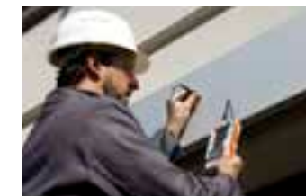
Measurement of anodizing coating on aluminum on a facade
